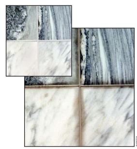
Studies show that all sealant chemistries can stain or cause streaking on porous substrates and glass and metal panels. *Dow Corning* 991 Silicone High Performance Sealant is specially formulated to resist dirt pick-up and prevent the fluid migration that can stain porous substrates and cause streaking on metal panels and glass.
